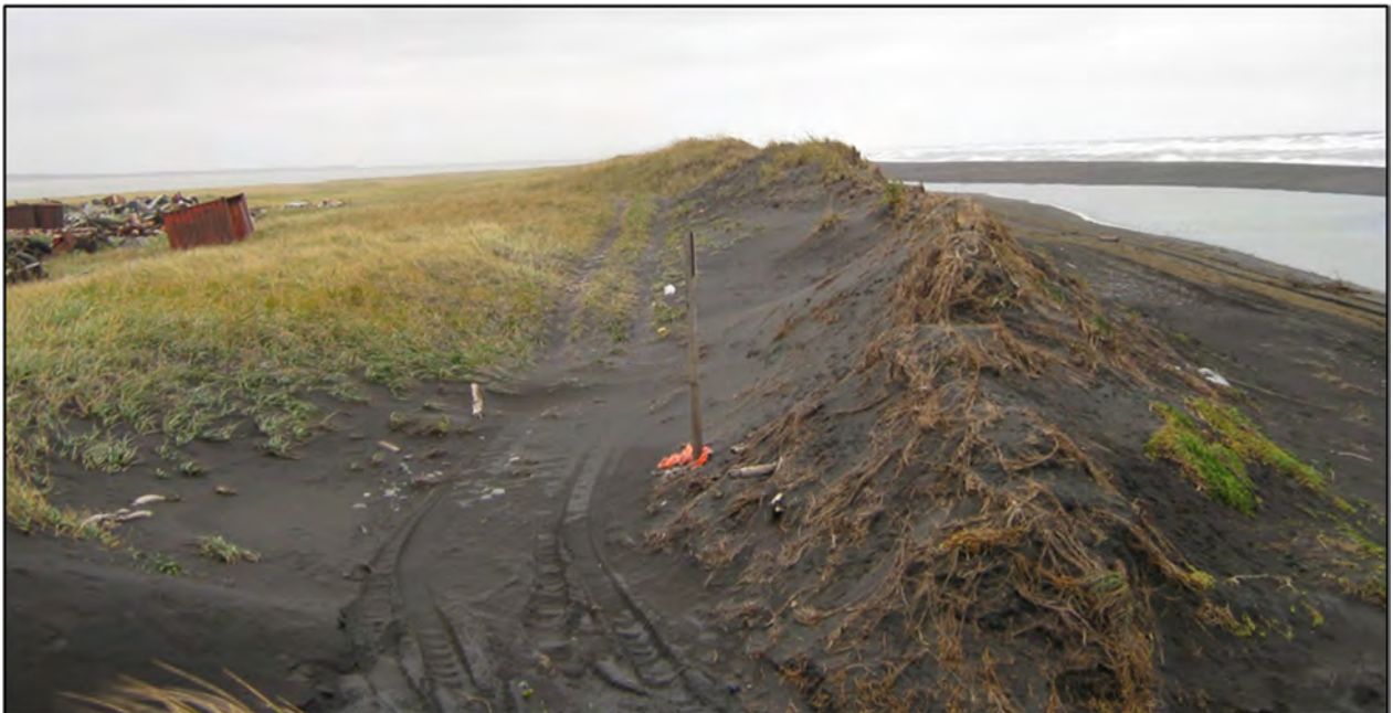
Figure 31. Remnants of an overwash and flooding event at the access road from the beach to the solid waste disposal site, October 2018 by UAF-ACGL.
